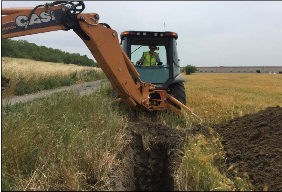
Photo 3: Test Pit WLCCB_08TP during excavation.
