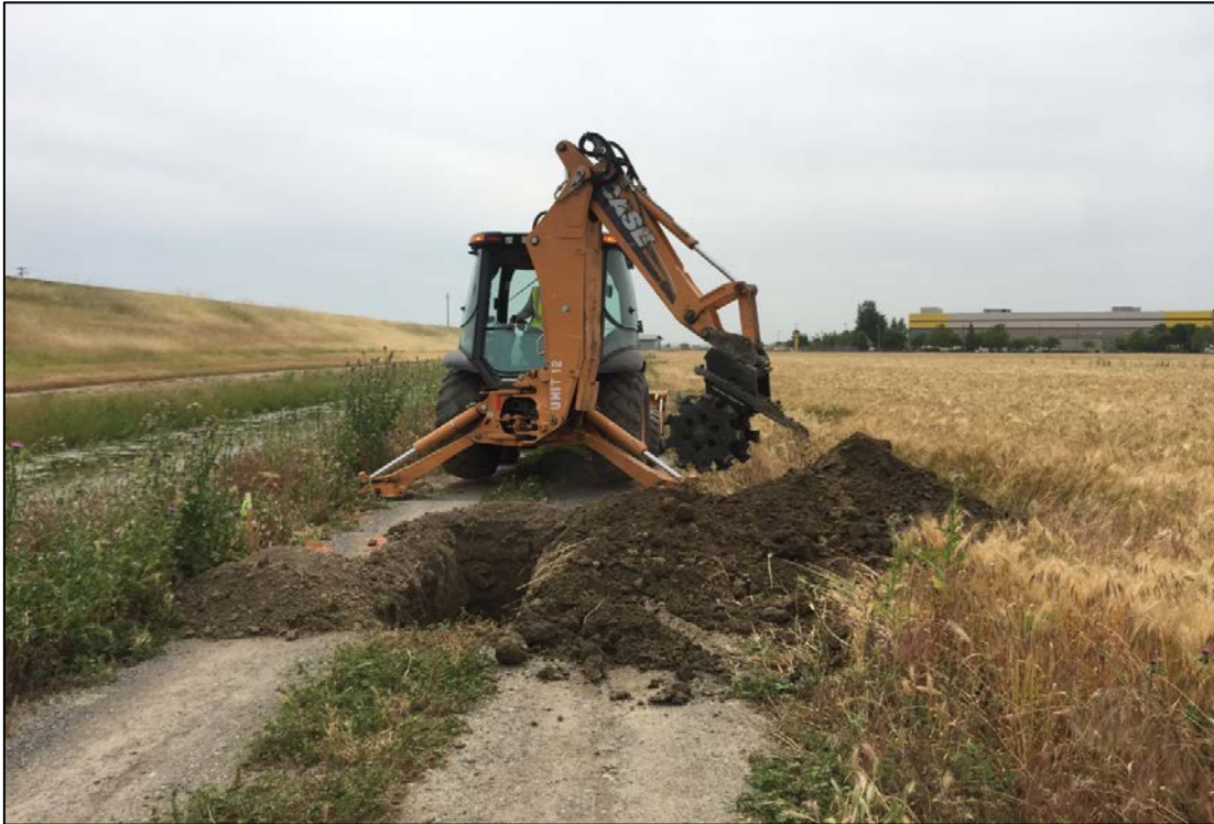
Photo 5: Test Pit WLCCB_09TP during excavation.
