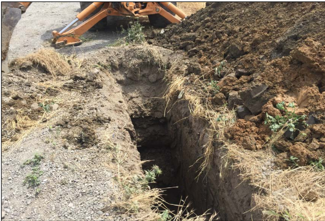
Photo 2: Test Pit WLCCB_09TP after excavation.
